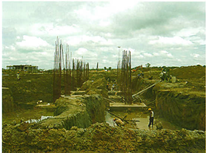
Piling work in progress at site
